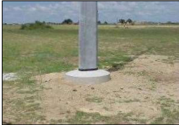
Plate 2: The base of the tower footing.
