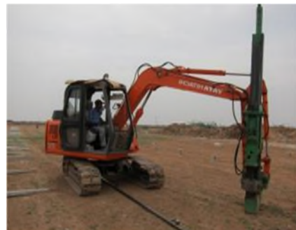
Pile Driving (Ram) Machine
