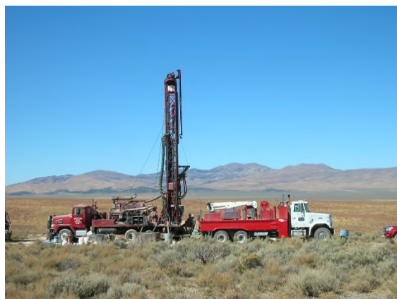
Picture 5 – Drill Rig
