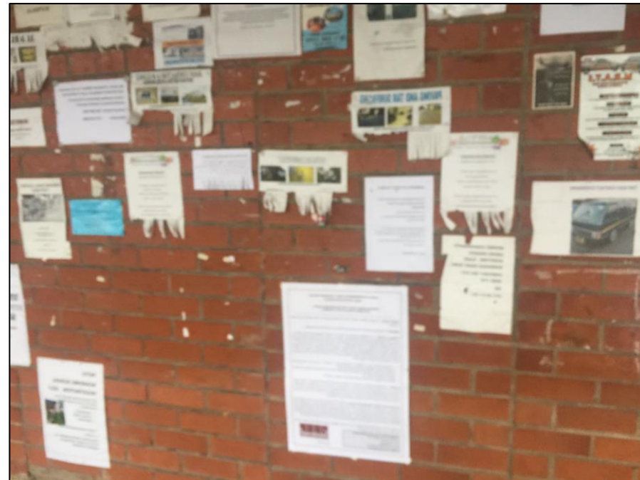
Full View of the site notice published on the notice wall of the Cato Ridge SPAR
