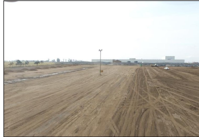
Wide Angle View of the Cato Ridge Facility
