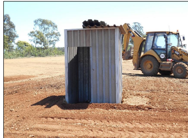
Guard Hut at the entrance to the site
