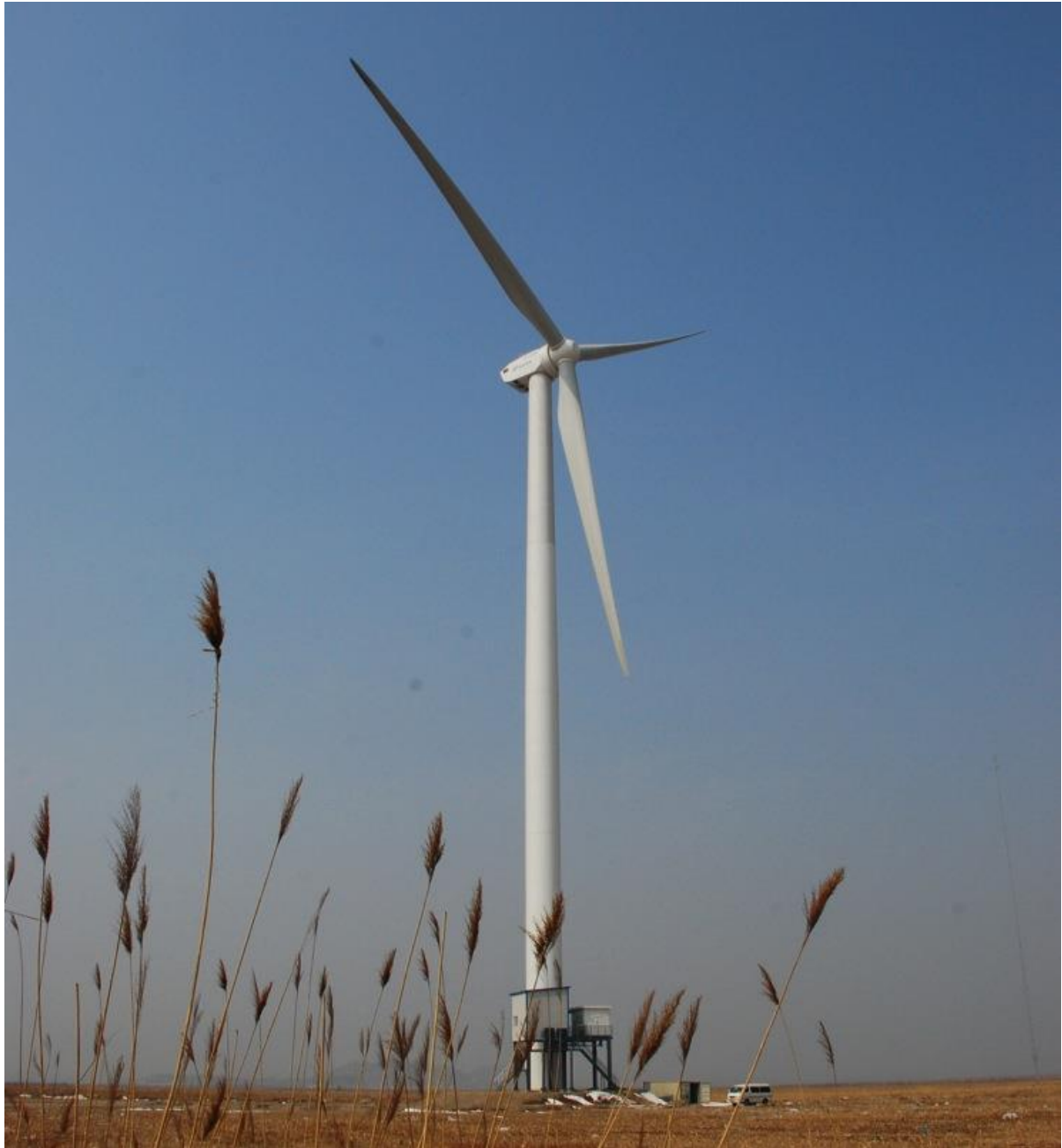
GW 2.5MW, Guanting Olympic Wind Farm
