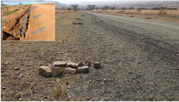
Figure 6-3 Example of road margin erosion prevention
